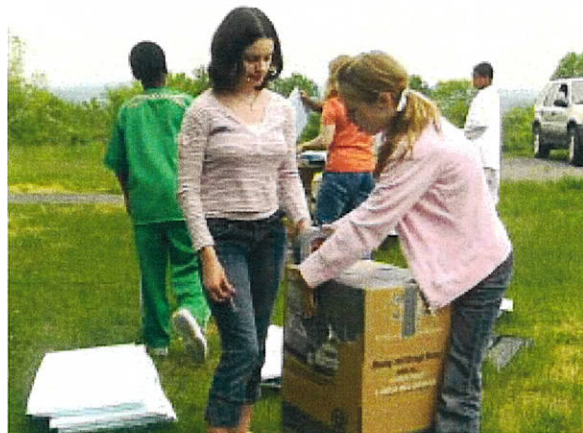
YES project middle-school students constructing a shelter for homeless cats as part of a unit on pet responsibility. The shelters were donated to an animal shelter and the students presented lessons on responsible pet care to elementary students.
